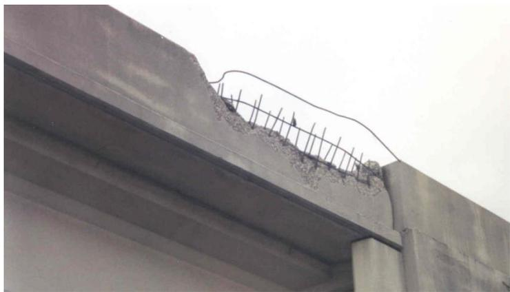
Figure 2. Damage to a 32" concrete bridge railing in a crash with a single unit truck in Florida. [Alberson04]
