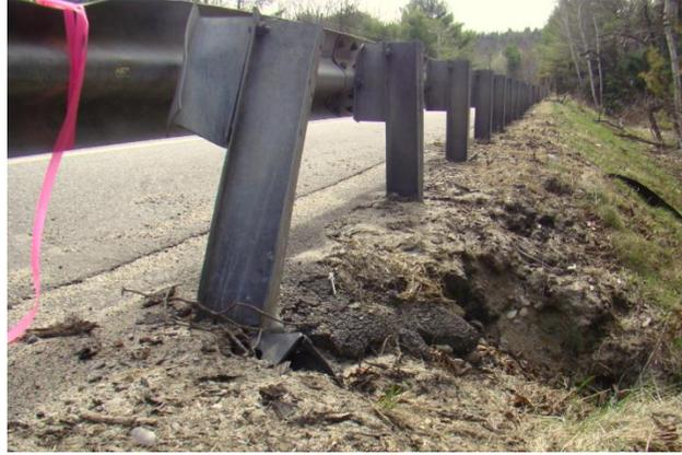
**Figure 1.** Example of soil erosion at a guardrail post.
